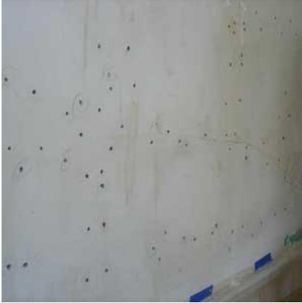
Drill holes on both sides of the cracks. If you miss lath, mark the holes with a pencil so you know not to put any adhesive in it.
