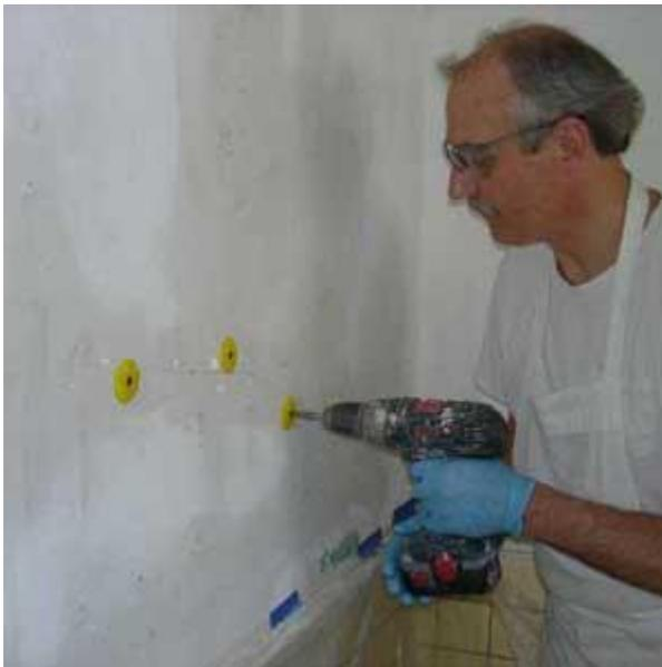
Screw plastic washers into a few of the holes to hold the lath against the adhesive until it sets. Remove the washers after a day or two, then fill the holes.
