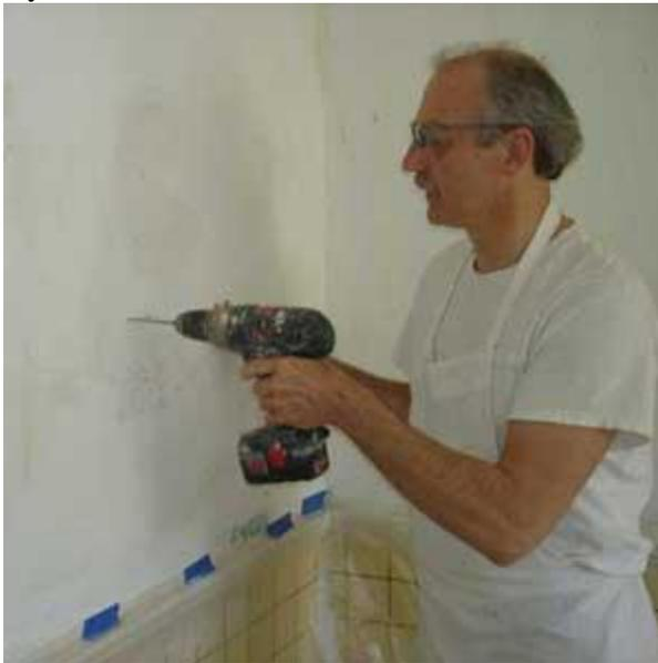
Using a 3/8-inch masonry bit, drill through the plaster on both sides of the crack. Stop drilling when you hit the wood lath.
